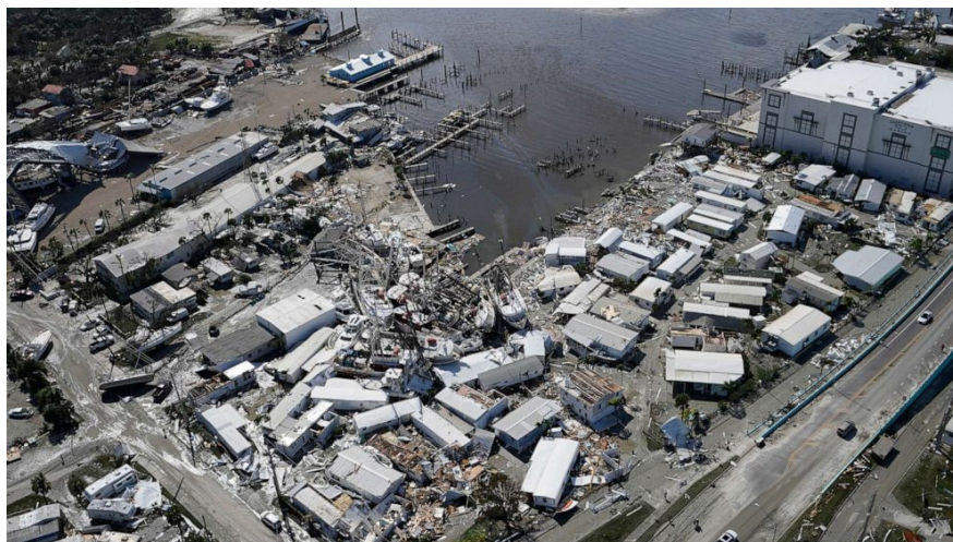
Figure 7. Hurricane Ian Damage on Captiva
