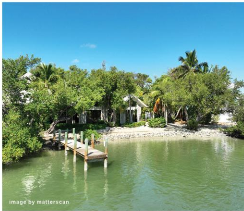
existing condition: residence proximity to water
