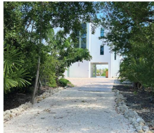
existing condition: low driveways prone to flooding
